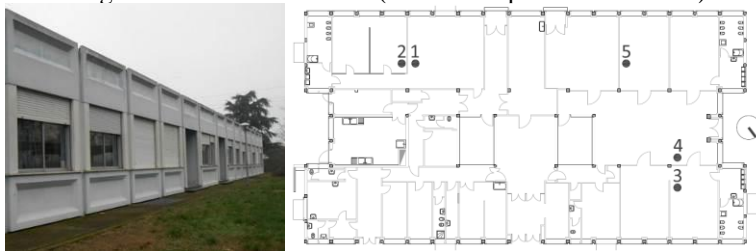
Fig. 1 (left) Picture of the southwest façade; (right) plan view with the five monitored rooms.
